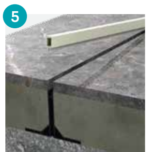
5 At least one day later the top hard plastic is removed.
